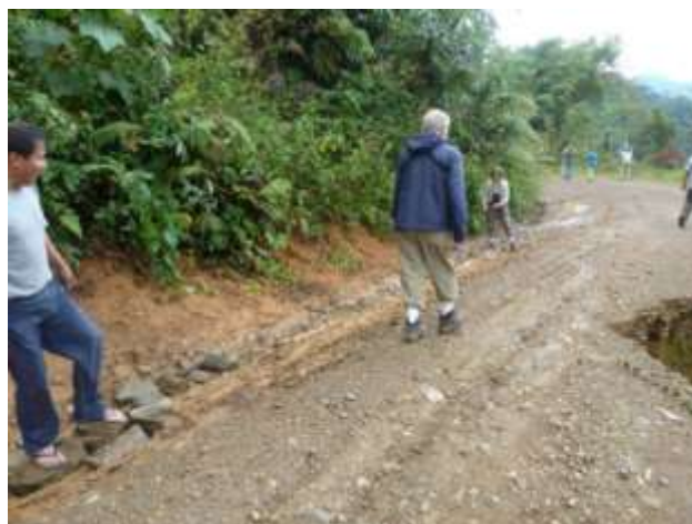
"Repairing" Manu Road
